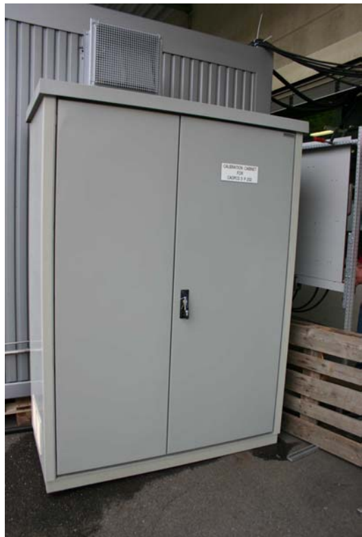
fiber glass cabinet for calibration gas cylinders
